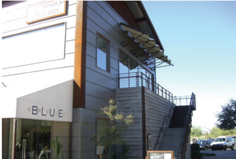
Carefully placed window canopies reduce energy consumption by providing shade in the summer while maintaining passive solar heating in the winter.
