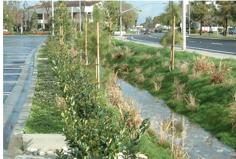
Routing stormwater into landscaped areas can reduce irrigation needs and enhance groundwater recharge.
