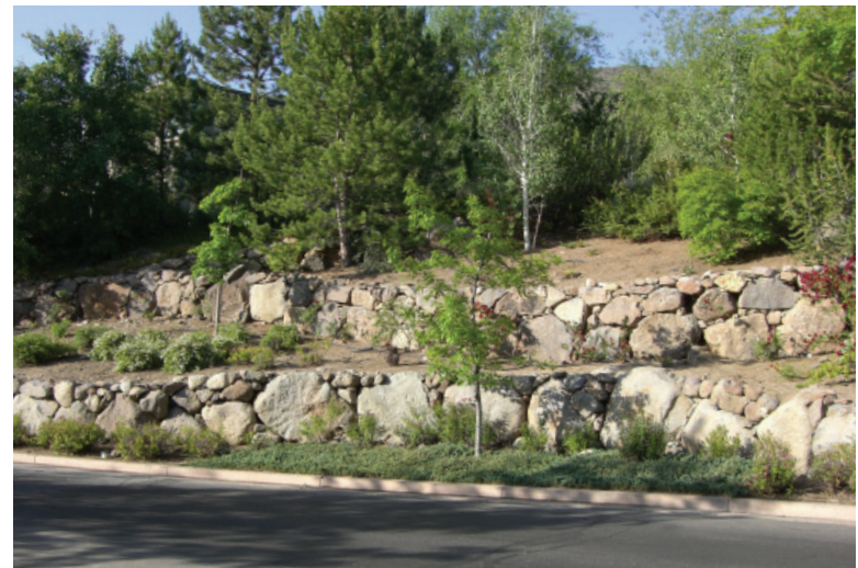
Meandering retaining walls and landscaping enhances community aesthetics.
