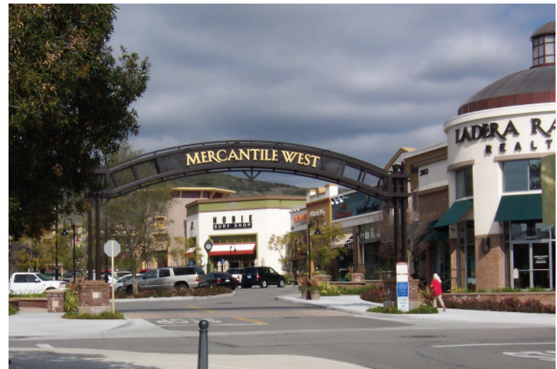
Entry features and other unique design elements help create a sense of arrival.
