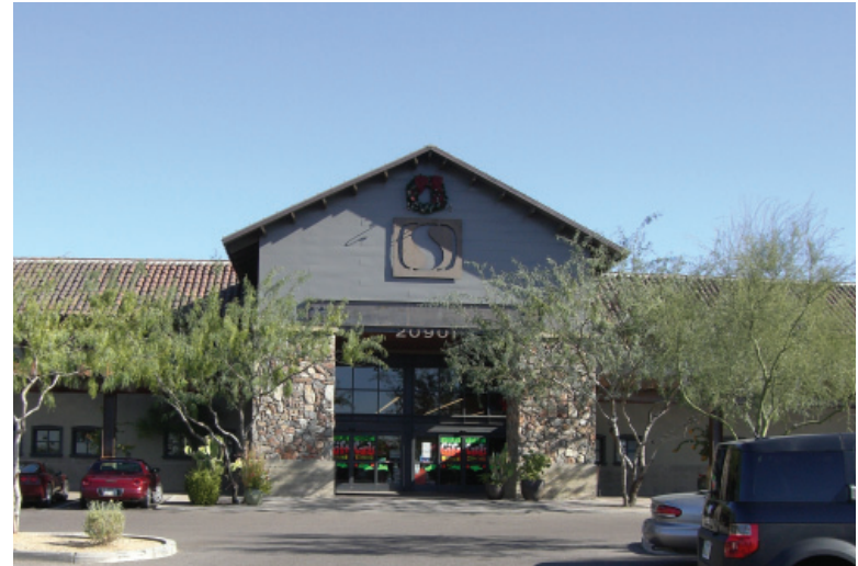
Signs should be compatible with building architecture.
